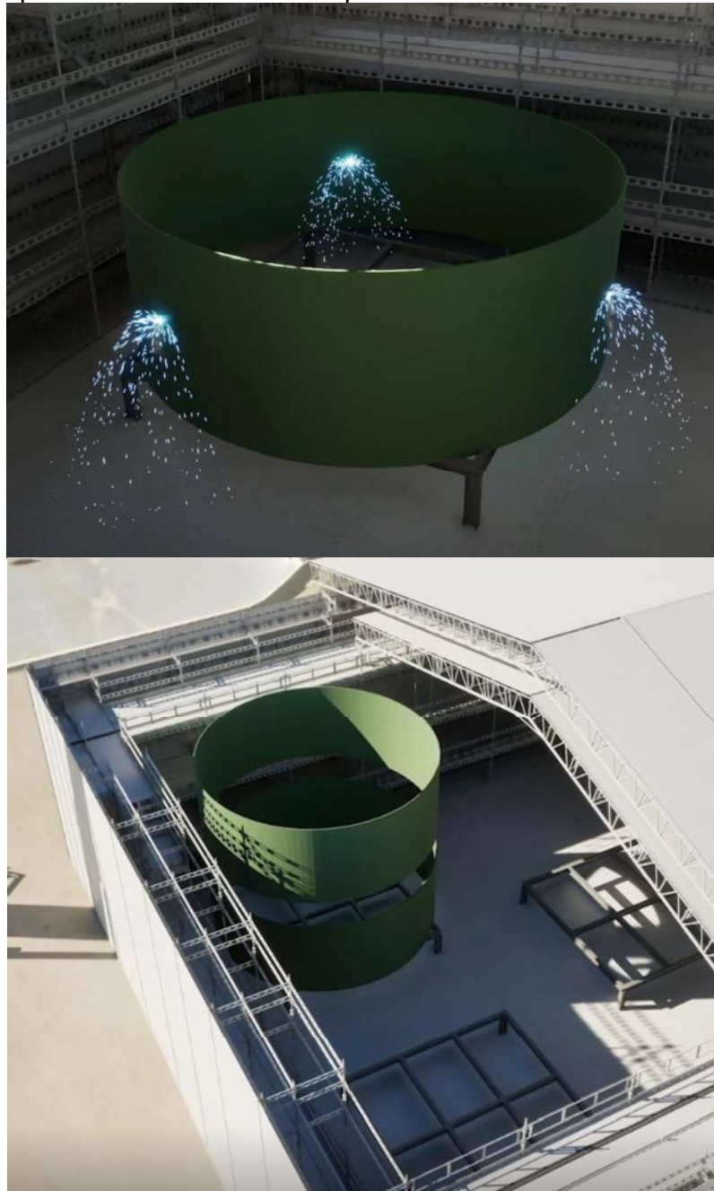
Figure 9-2 Typical Prefabrication of Absorber at Site
