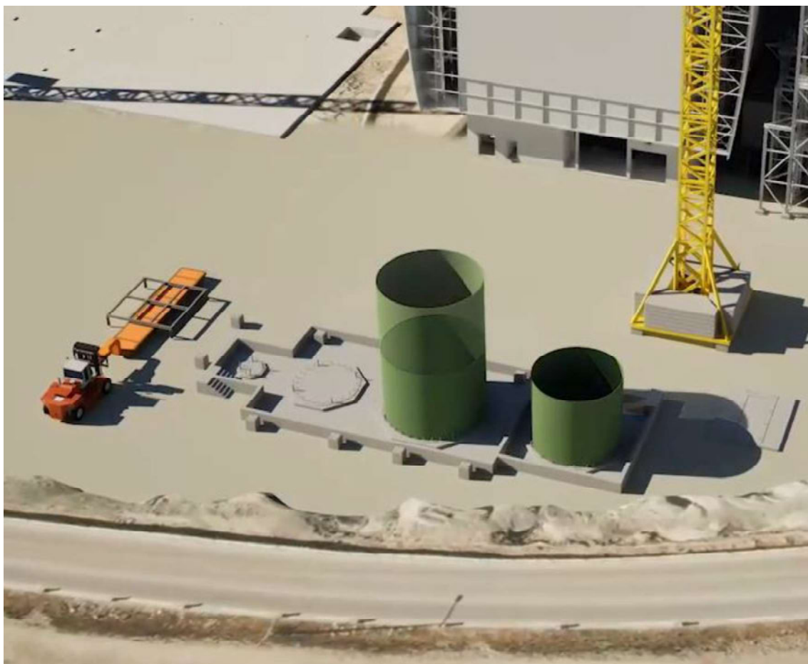
Figure 93 Assembly of Absorber / DCC
