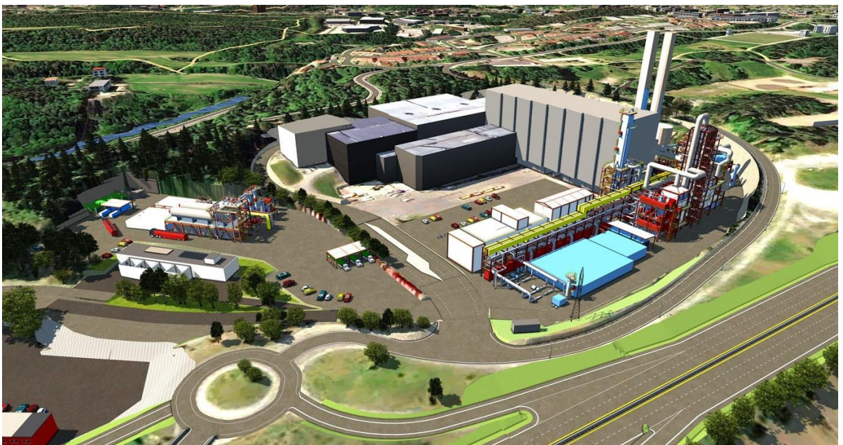
Hafslund Oslo Celsio's CO 2 capture plant will be capturing 400 000 tonnes of CO 2 from 2026.
