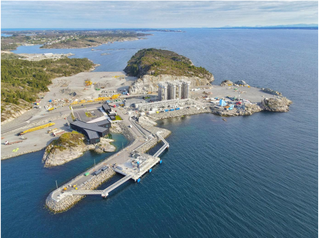
Northern Lights' CO 2 receiving terminal in Øygarden.
