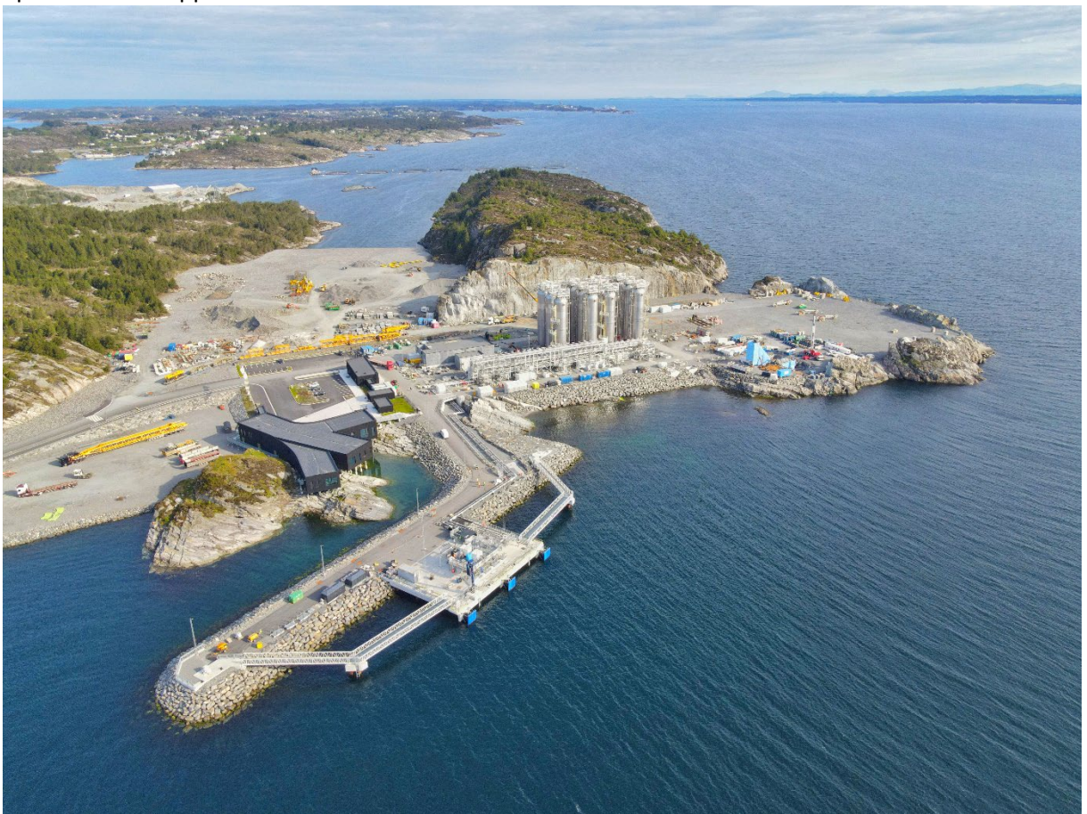
Northern Lights' CO 2 receiving terminal in Øygarden.
