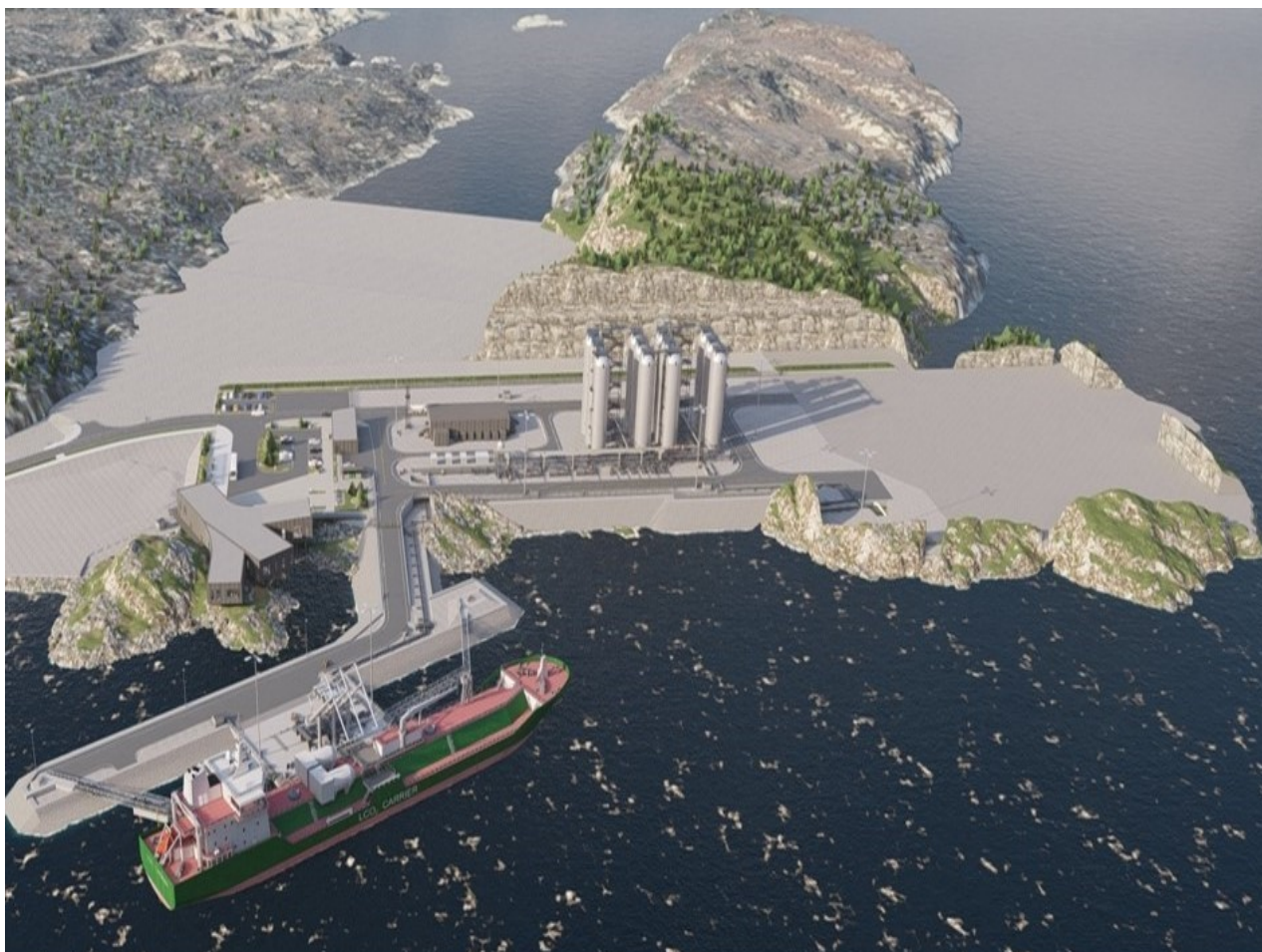
Northern Lights' CO 2 receiving terminal in Øygarden.
