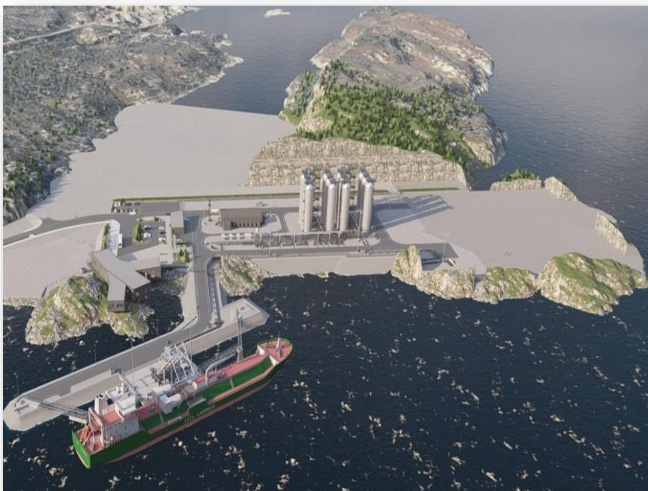
Northern Lights' CO 2 receiving terminal in Øygarden.
