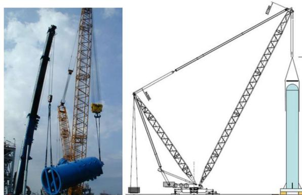
Figure 56 - Handling of large columns/ tanks including up-ending
