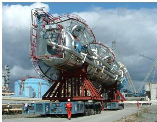
Figure 55 - Use of SPMT - Reference picture from Kårstø
