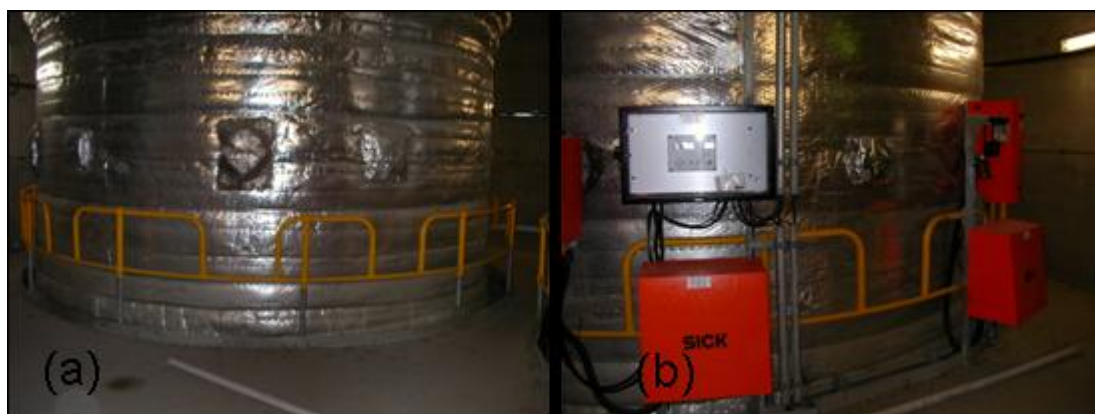
Figure 2.14. An example of the well designed and positioned sampling points within the stack shown in Figure 2.13: (a) sample ports visible; (b) online gas analysers installed in sample plane. (Copyright CSIRO, CCSD 2010)
