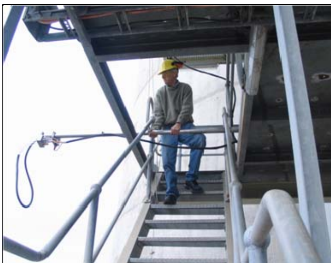
Figure 2.12. Example of poorly designed work platform. *
