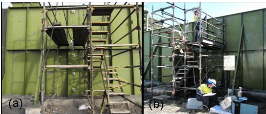
Figure 2.9. Temporary scaffolding used to support personnel support while sampling: (a) scaffolding treads were removed to enable measurements whereas in (b) horizontal scaffolding structural sections were remove to allow sampling probe insertion. (Copyright CSIRO 2010)
