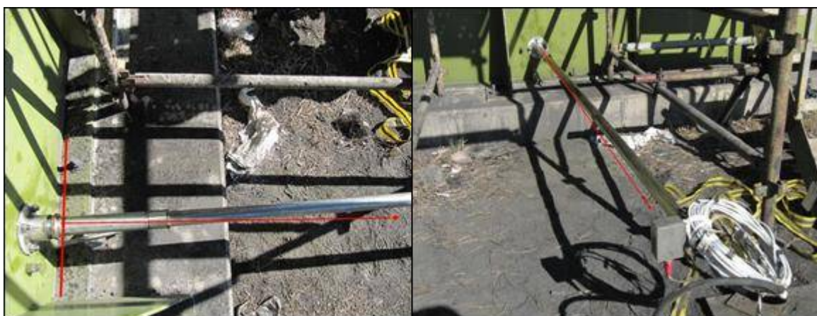
Figure 3.4. An example of misalignment of a sampling port access flange. (Copyright CSIRO 2010)
