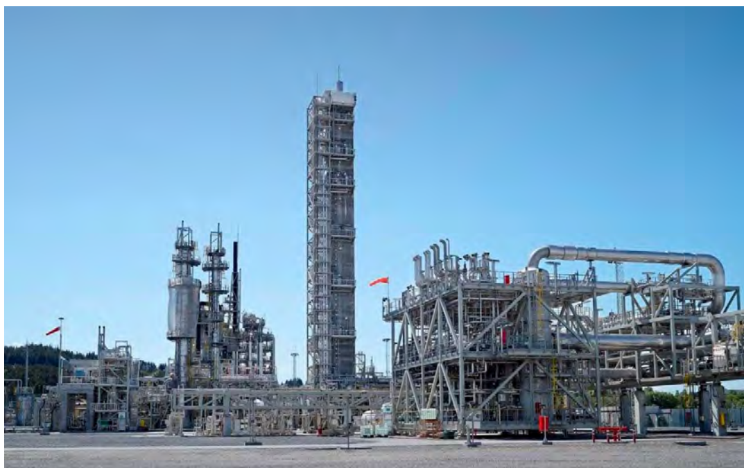
Fig. 2. TCM DA amine plant. The direct-contact cooler is situated to the right, the concrete absorber tower in the middle, the two stripper columns to the left, and the lean vapour compressor system to the far left.
