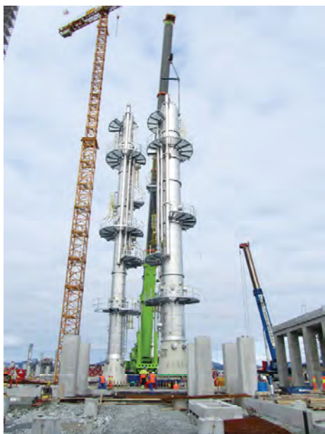
Figure 1 Picture of final placement of the two desorbers
