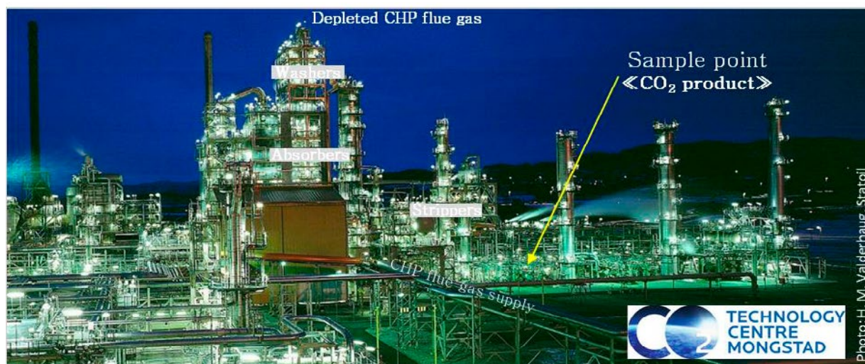
Fig. 1. Technology Centre Mongstad (TCM), Norway [Photo © Equinor] DA amine plant with CHP flue gas inlet from the front, and the high absorber tower in the middle. "Captured" CO 2 product outlet and sample point towards the right.
