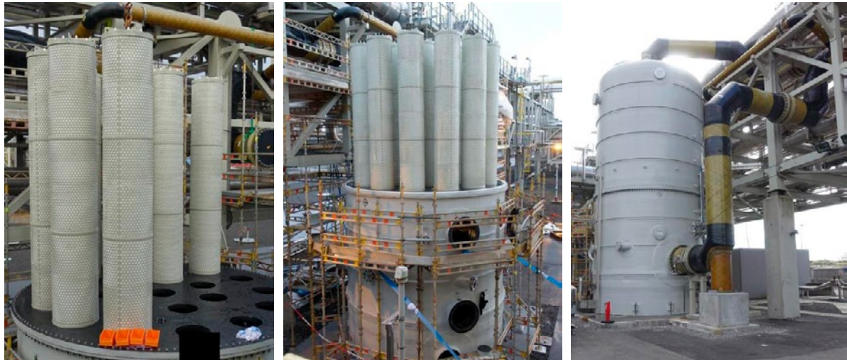
Figure 3 Installation pictures. To the left: main support plate of the candles. To the right: the flue gas inlet is located at the bottom of the vessel.
