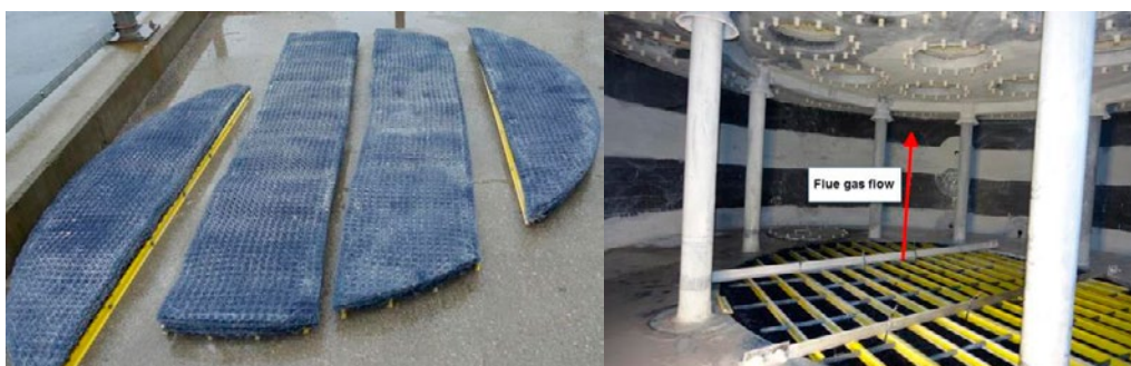
Figure 5. High efficiency demister. To the left: demister pads disassembled for cleaning operation. To the right: the demister pads are located under the yellow support grid. The candle support plate with the openings to the candles is visible at the top of the picture.
