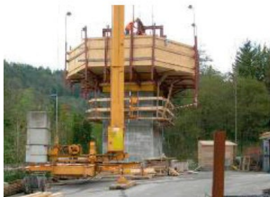
Figure 6 Picture of slip forming mock-up with actual design and dimensions of concrete absorber with liner
