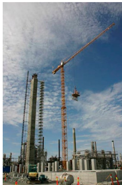
Figure 2 Picture of construction of the amine unit with finalized slip formed absorber
