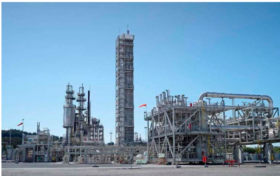
Fig. 2. TCM DA amine plant. The direct-contact cooler is situated to the right, the concrete absorber tower in the middle, the two stripper columns to the left, and the lean vapor compressor system to the far left. The platforms towards the upper part of the absorber towers indicate the access location for the sample ports for the aerosol measurements.
