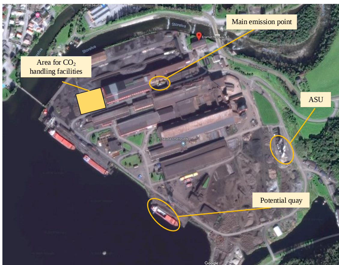
Figure 14. Overview of the Eramet Sauda plant and surroundings (© Google Maps).
